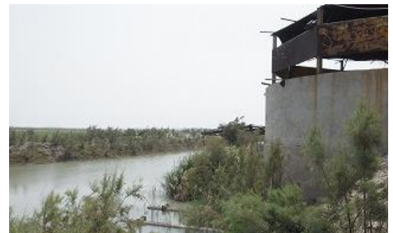
4 - Existing intake facility
