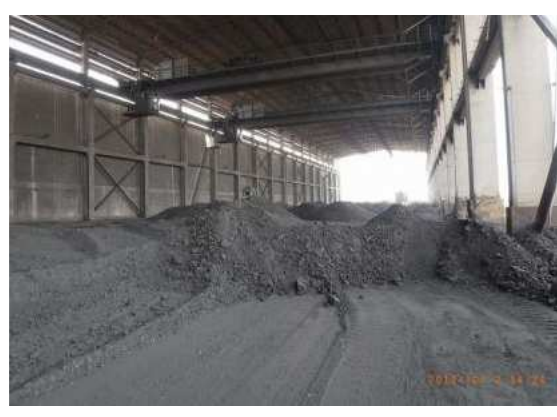
Existing Coal Storage
