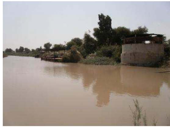
Water Intake Site
